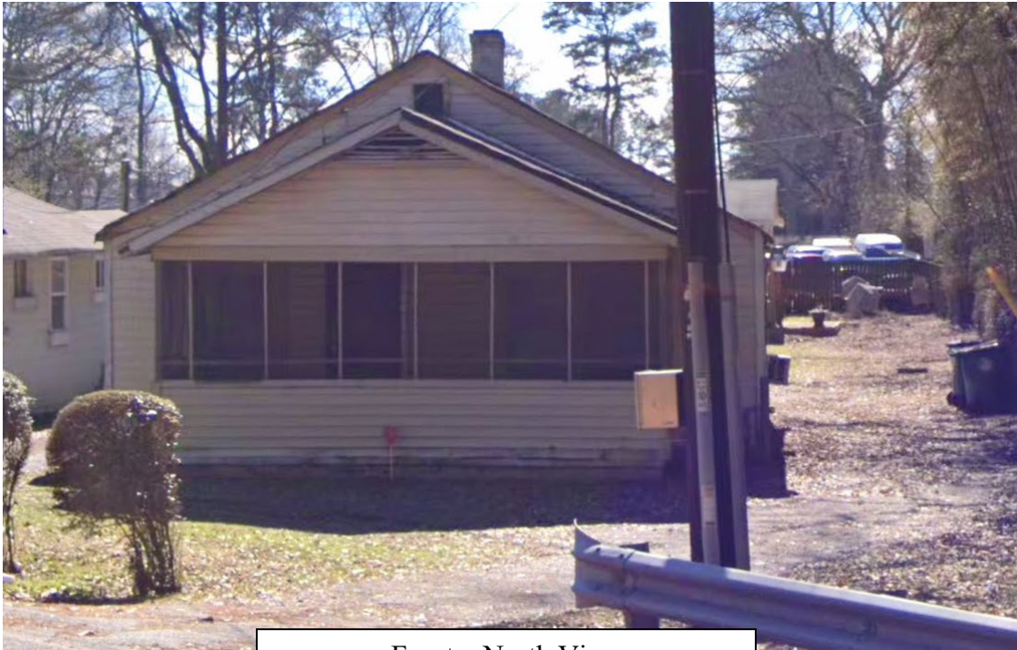
Front – North View
