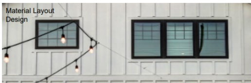
Exterior Siding: Board and Batten
