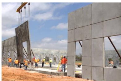
Exterior Siding: Concrete Tilt Panel
