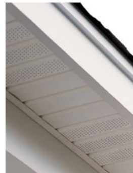
Soffit: Vinyl Soffit, Metal Wrap Fascia
