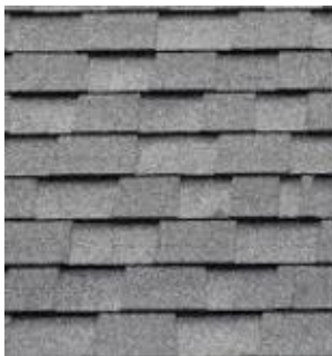
Roof: Architectural Shingles
