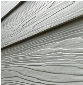
Exterior Siding: Fiber Cement Siding
