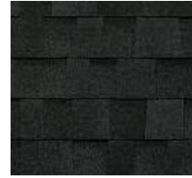
Roof: Asphalt Shingles (Black)
