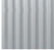
Secondary Roof: Galvanized Metal Roof
