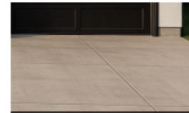
Natural Gray Concrete Concrete Elements Porch/Driveway/Steps
