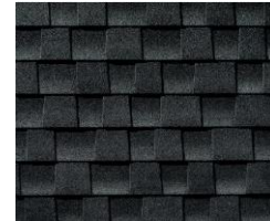
Roof: Architectural Shingles (Black)
