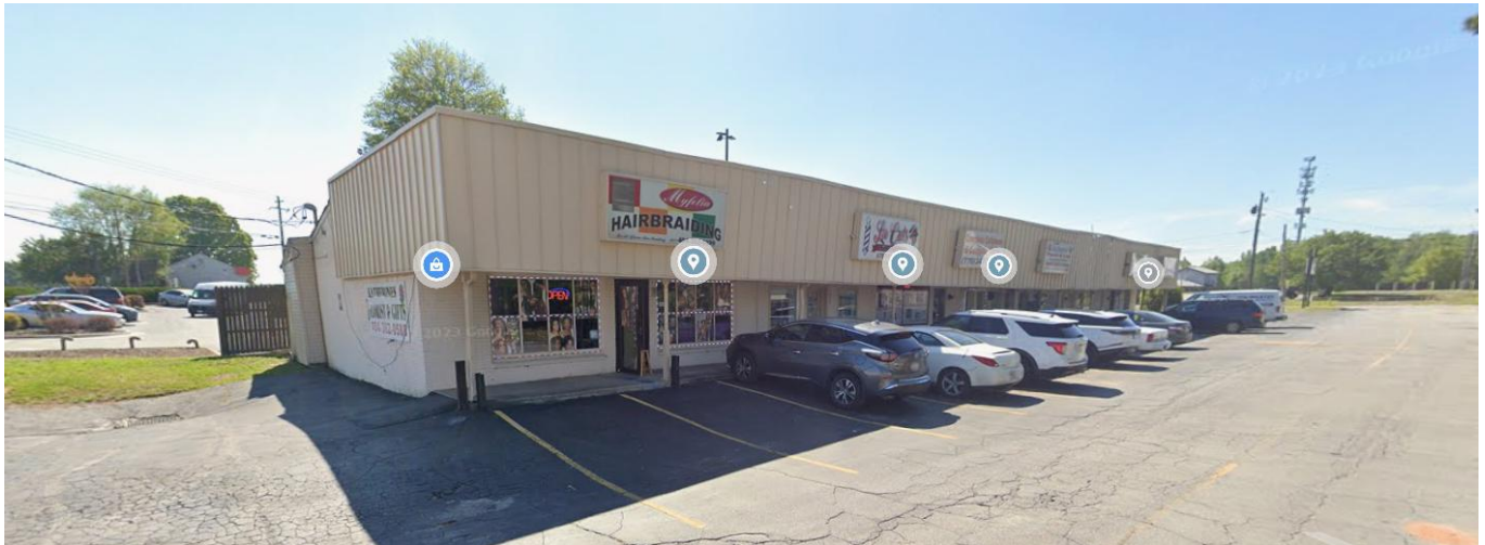
Site prior to damage on metal fascia
