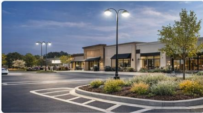
UPGRADED PARKING LOT LIGHTING
