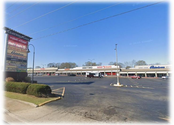
Existing Conditions: Clayton Plaza
